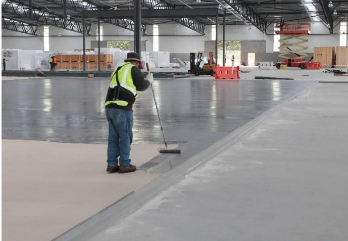
Application of Ucrete DP in the beer processing area and packaging room
