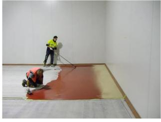
The concrete slab floor was first shot-blasted and had minor repairs made, prior to a 9mm thick trowel application of Ucrete DP20
